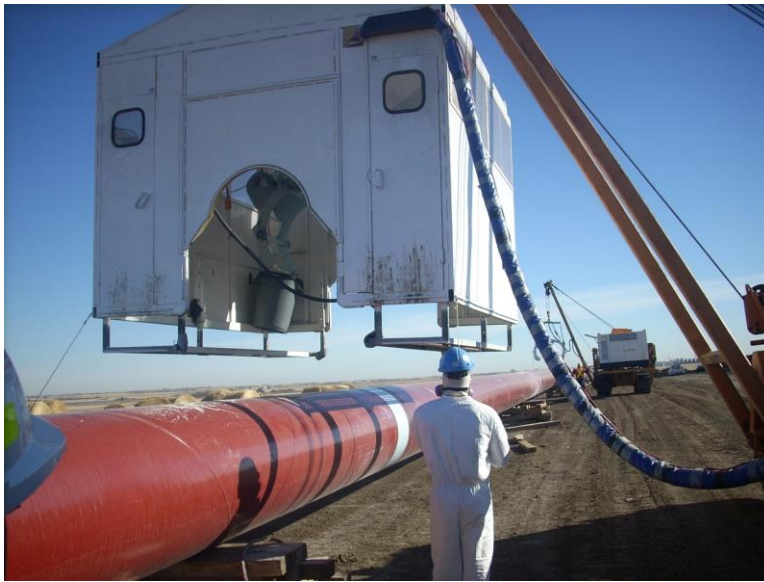
Girth Weld Coating Shack
