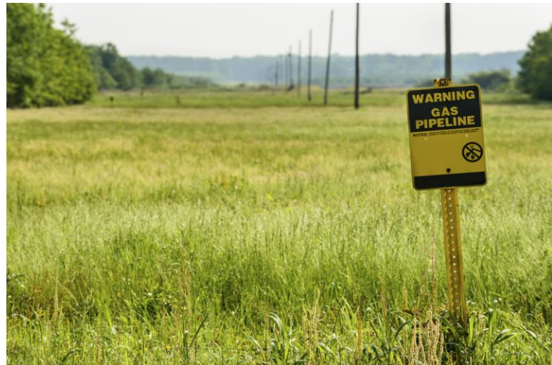
Marker indicating a buried pipeline
