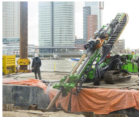
Horizontal Directional Drilling (HDD)
