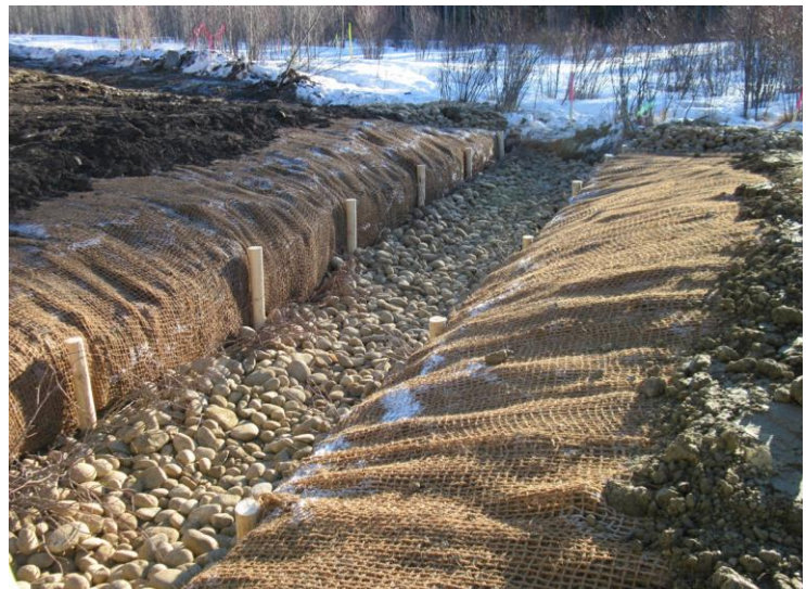
Isolated Trench Crossing
