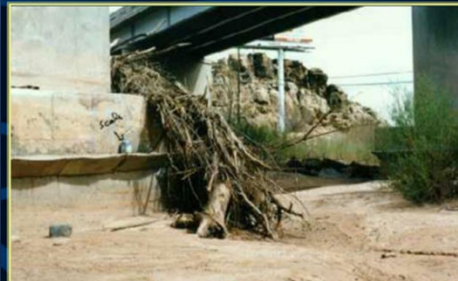
Field Evidence Of Long-Term Scour
